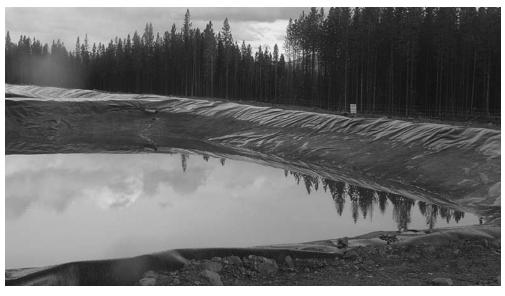
Coalbed methane produced water treatment pit near Fernie. Note iron oxide residue on the plastic liner.
