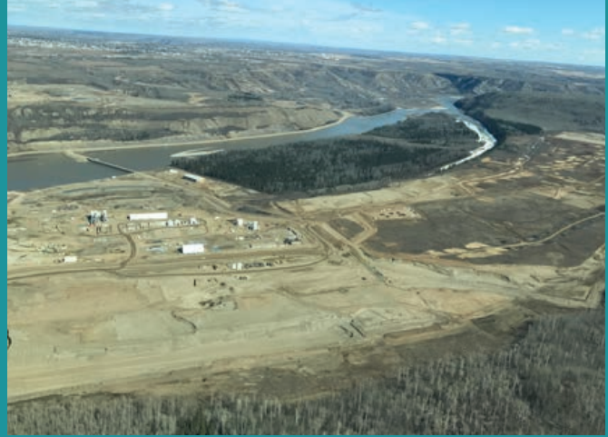
Site C construction, 2017
